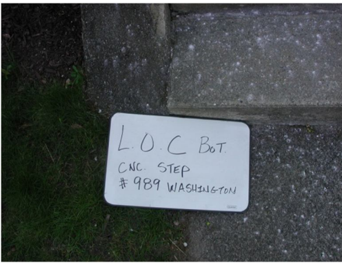
BM LOCBCS 989 ~ Left Outer Corner Bottom Conc. Step @ HSE. #989 Washington St.
