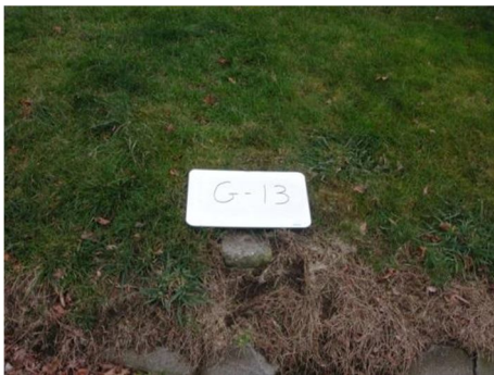
BM G13 Drill Hole Stone Bound.
