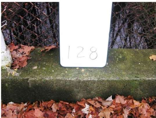
BM 128 Brass Rivet on top of Concrete Headwall.
