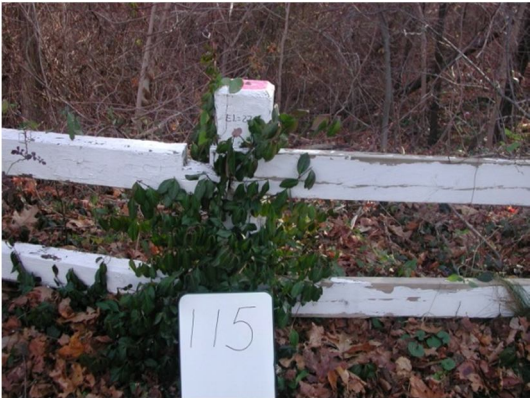
BM 115 Brass Rivet on top of Concrete guard rail post.
