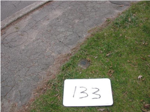
BM 133 Disk on top of Concrete Bound.
