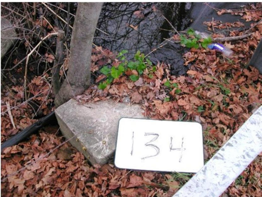
BM 134 Brass Rivet on top of Concrete Headwall.
