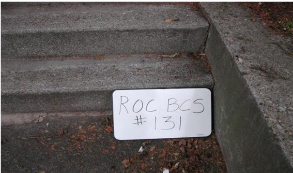
BM ROCBCS 131S ~ Right Outer Corner Bottom Conc. Step @ HSE. #131 Summer St.
