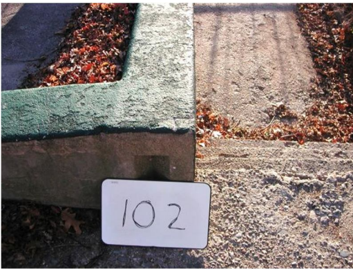
BM 102 Square Cut on top of Concrete Retaining wall to Parking Area @ Wessagussett Rd..
