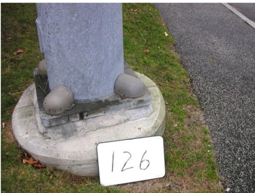
BM 126 Brass Rivet on top of Concrete Pier of Traffic Pole.
