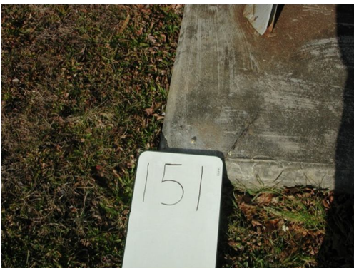
BM 151 Brass Rivet on top of Concrete pad.
