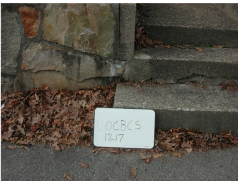
BM LOCBS 1217 ~ Left Outer Corner Bottom Conc. Step @ HSE.#1217 Commercial St.
