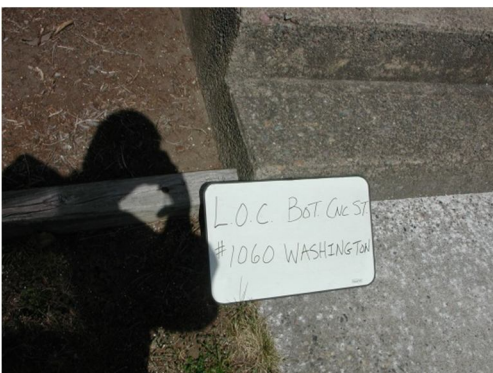
BM LOCBCS 1060 ~ Left Outer Corner Bottom Conc. Step @ HSE. #1060 Washington St.
