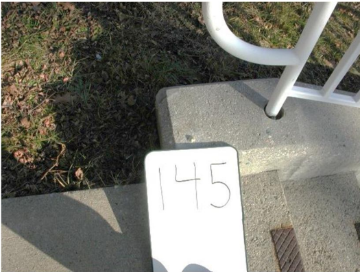
BM 145 Brass Rivet on top of Concrete retaining wall for stairs.
