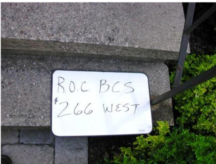
BM ROCBCS 266 ~ Right Outer Corner Bottom Conc. Step HSE. #266 West St.
