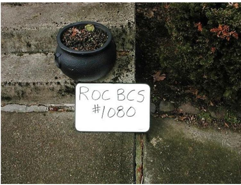
BM ROCBCS 1080 ~ Right Outer Corner Bottom Conc. Step @ HSE. #1080 Pleasant St.
