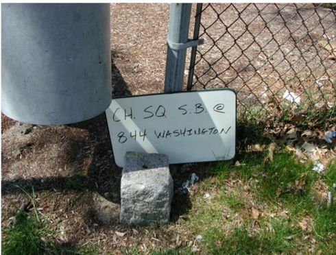
BM CHSQRBS 844 ~ Chiseled Square Cut Stone Bound @ HSE. #844 Washington St.
