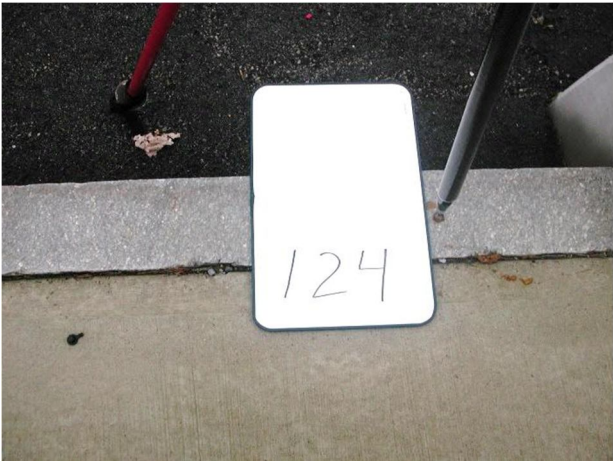
BM 124 Brass Rivet on top of Granite Curb.
