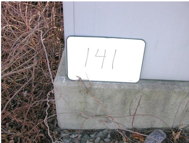
BM 141 Square Cut on top of Concrete Base.
