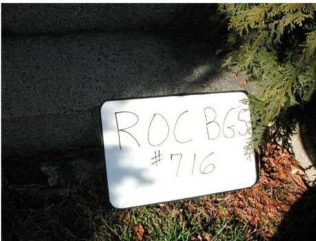
BM ROCBGS 716 ~ Right Outer Corner Bottom Granite Step @ HSE. #716 Commercial St.
