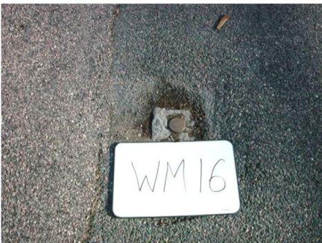
BM WM16 Disk on top of Granite Bound.
