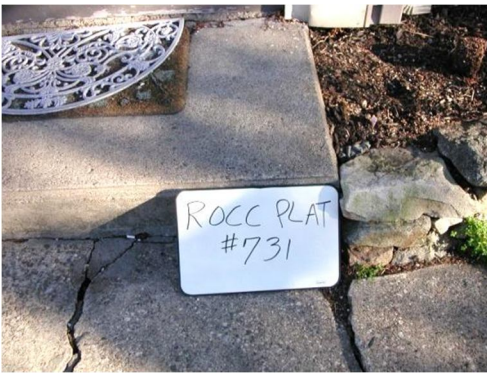
BM ROCCPL 731 ~ Right Outer Corner Conc. Platform @ HSE.#731 Pleasant St.
