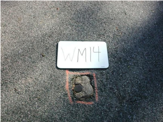
BM WM14 Disk on top of Granite Bound.
