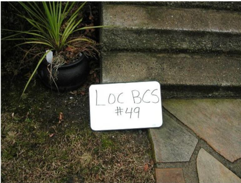
BM LOCBCS 49 ~ Left Outer Corner Bottom Conc. Step @ HSE. #49 Pleasant St.
