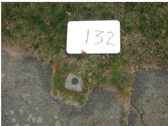
BM 132 Disk on top of Concrete Bound.
