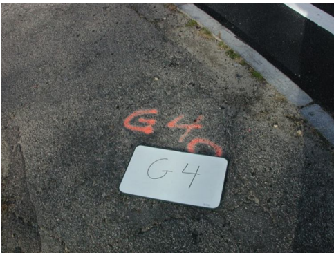
BM G4 Spike in bitumimous Concrete Pavement.
