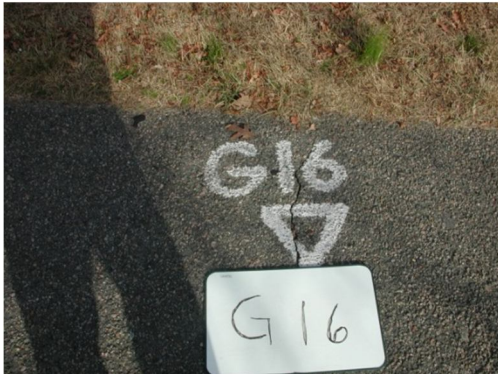
BM G16 Spike in bituminous Concrete pavement.
