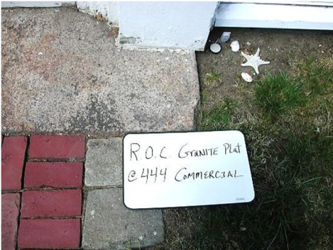
BM ROCGPLAT 444 ~ Right Outer Corner granite Platform @ HSE. #444 Commercial.
