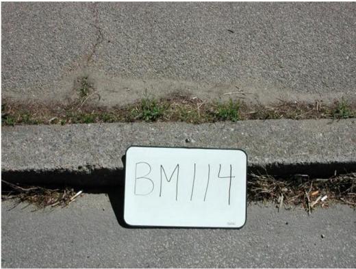
BM 114 Rivet on top of Concrete curb.
