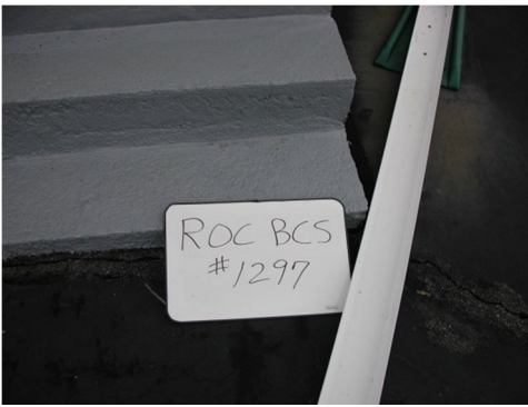
BM ROCBCS 1297 ~ Right Outer Corner Bottom Conc. Step @ HSE. #1297 Pleasant St.
