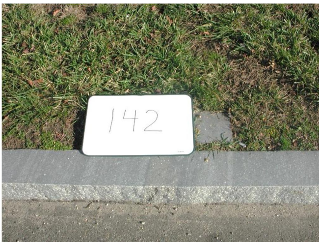
BM 142 Brass Rivet on top of Granite Bound.
