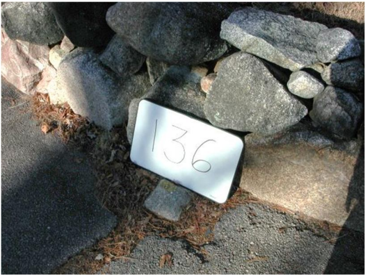
BM 136 Brass Rivet on top of Concrete Bound.
