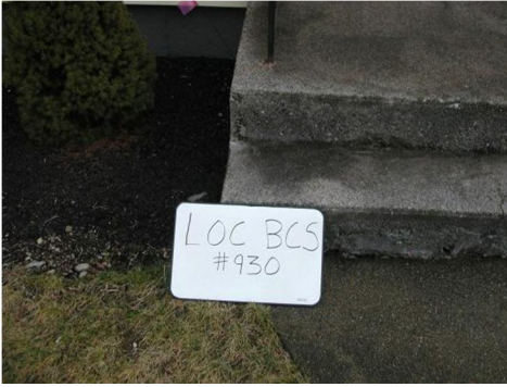
BM LOCBCS 930 ~ Left Outer Corner Bottom Conc. Step @ HSE. #930 Middle St.
