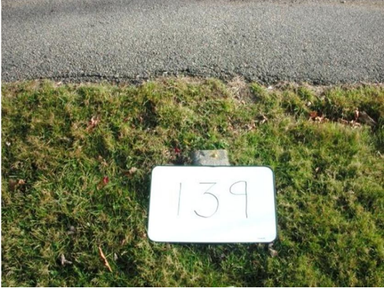
BM 139 Brass Rivet on top of Concrete Bound.
